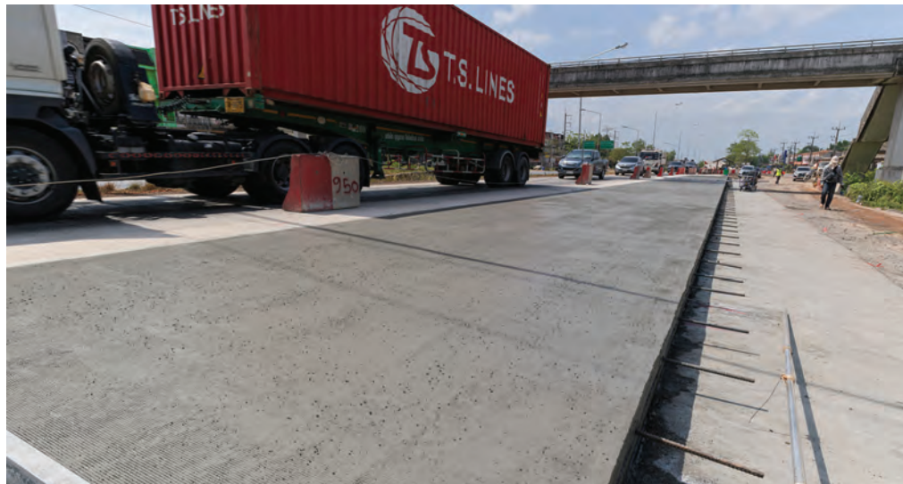
TOP AND ABOVE: Premium Concrete deploys a Wirtgen SP 64 slipform paver for the construction of a 22.3-km-long road in Surat Thani.
