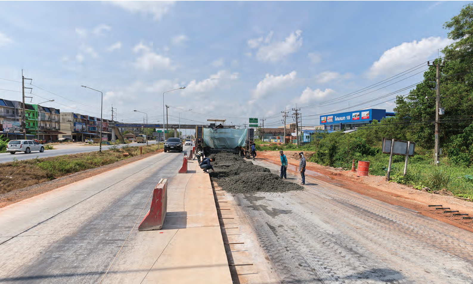
ABOVE AND BELOW: The new road section in Surat Thani has an overall width of 11 m, with two 3.5-m lanes and one 4-m lane. The SP 64 slipform paver enables an extremely even, high-quality concrete surface.
