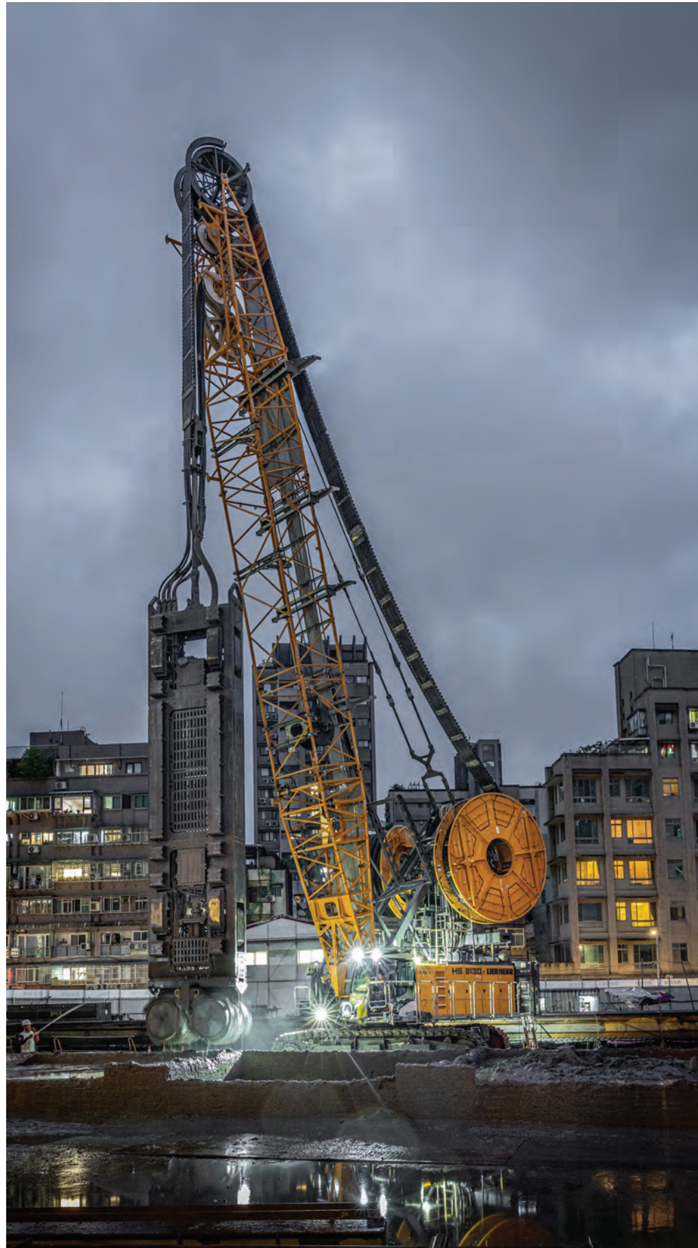
Using the LSC 8-18 slurry wall cutter, Tung Feng was able to advance at an average of 4 m per hour. The finished slurry walls reached down to depths of 30 to 55 m and were between 800 and 1,500 mm thick.
