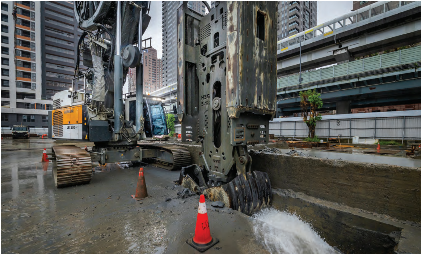
ABOVE AND BELOW: The standard version of the LBX 600 carrier machine features a total height of 17.8 m. For operations with limited headroom, work can be carried out in low-head configuration at 11 m or ultra-low-head configuration at 5.8 m.
