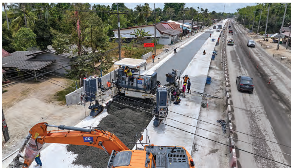
TOP, MIDDLE AND ABOVE: The Wirtgen SP 64 slipform paver also helps CC Machinery & Construction upgrade a 17-km road section in Tha Sala.
