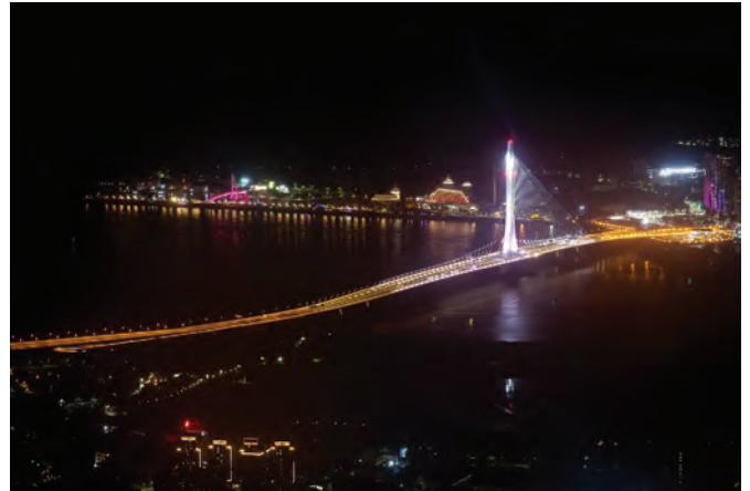
The opening of the Danjiang Bridge marks a major milestone for Taiwan after nearly three decades of planning and construction. This new bridge serves as a regional transport link connecting the Tamsui and Bali districts.
