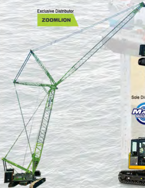
Crawler Crane with luffing jib
