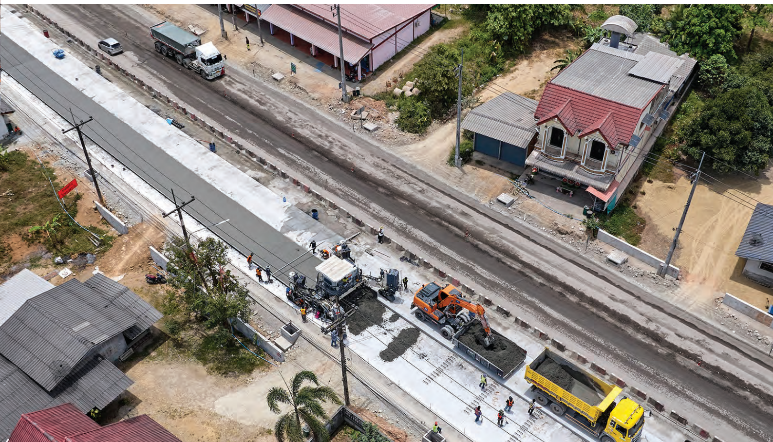
ABOVE AND BELOW: The upgraded road in Tha Sala is 14 m wide overall, with four 3.5-m lanes. It features a concrete surface thickness of 25 cm on the right and 28 cm on the left.
