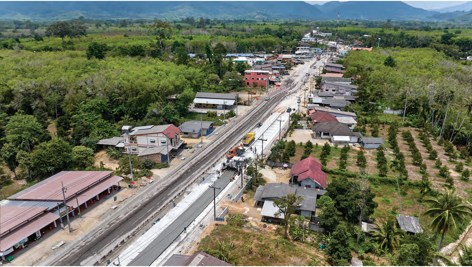
ABOVE AND BELOW: The upgraded road in Tha Sala is 14 m wide overall, with four 3.5-m lanes. It features a concrete surface thickness of 25 cm on the right and 28 cm on the left.
