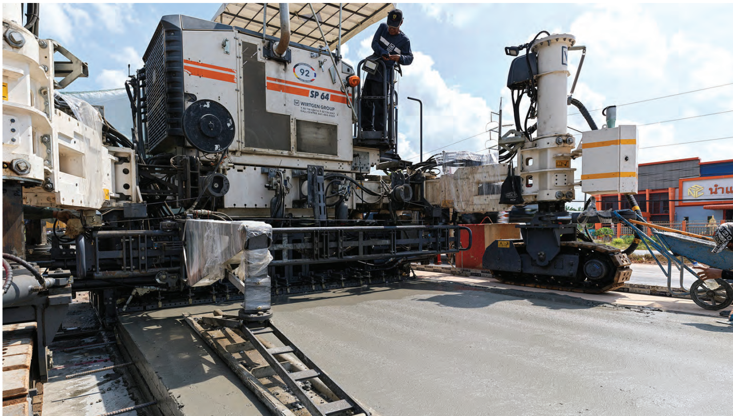
ABOVE AND BELOW: The new road section in Surat Thani has an overall width of 11 m, with two 3.5-m lanes and one 4-m lane. The SP 64 slipform paver enables an extremely even, high-quality concrete surface.
